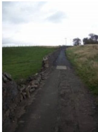
End of new surface at broken wall section
